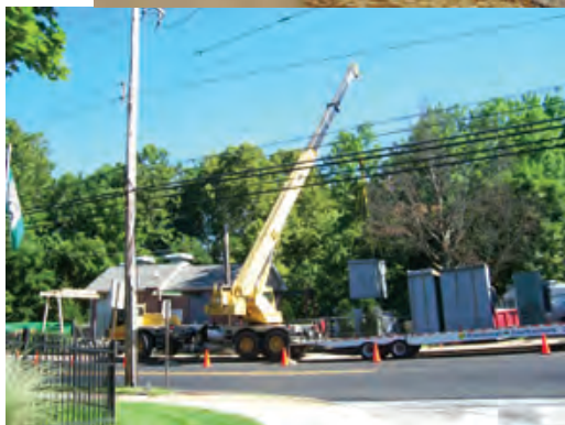
Bottom photo shows the pump station's old transformer and switchgear being removed and loaded.
