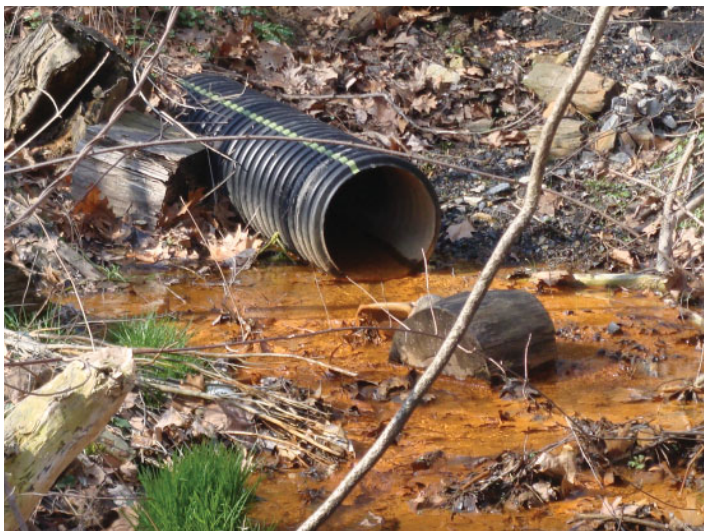
Bright orange water coming from the piping clearly shows high levels of iron.
