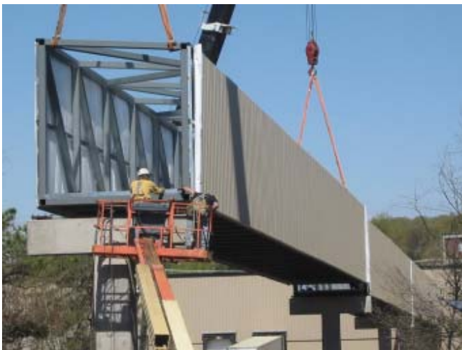
Setting bridge section on bearing plates
