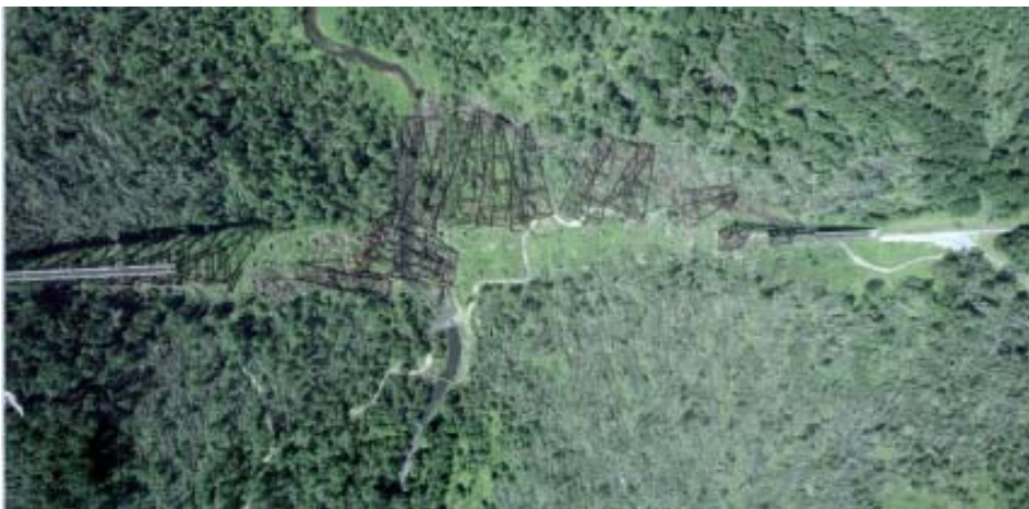
Aerial photography of the Kinzua site was crucial in determining the cause and order of collapse
