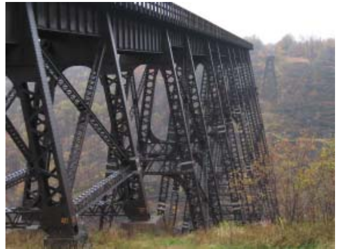
The Kinzua Viaduct — October 2004
