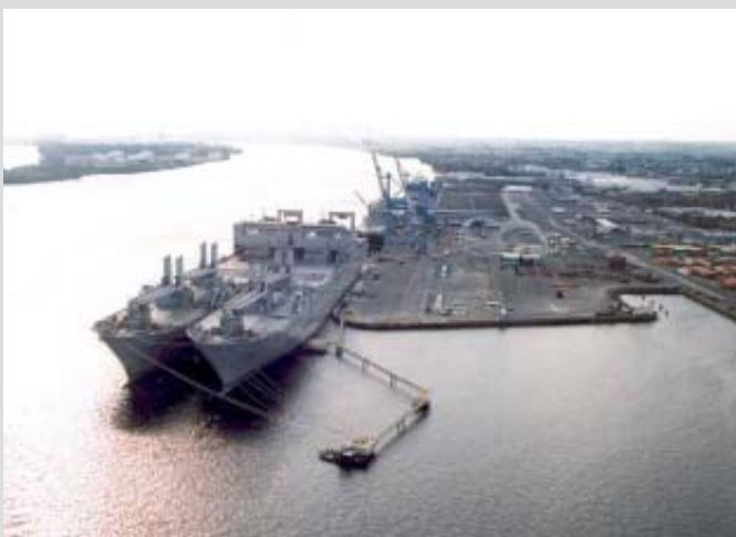
Overall View of the Berth with LMSRs Moored
