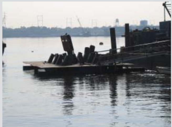
Falsework for the Breasting Dolphin Pile Installation
