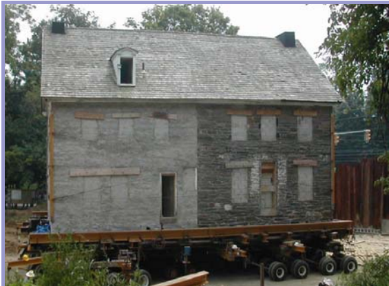
During the move, Rose Tree Tavern sat on 20 sets of dollies, each with 8 wheels. The air in all 160 super-size tires had to be checked before the Tavern could be broken free from its foundation.
